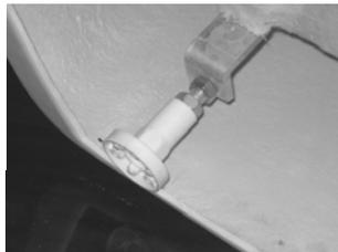
2. Using a spirit level check to ensure the top edge of the bath is level. If necessary use the levelling feet to adjust. Adjusting the feet will cause the acrylic surround to lift off the floor.
