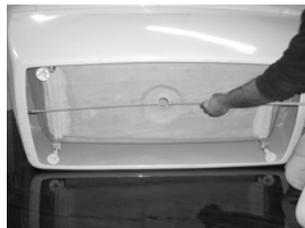
4. Connect the waste and lower the bath into position.
